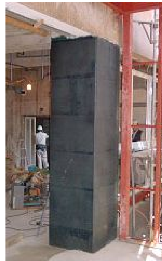
Pillar reinforcement
