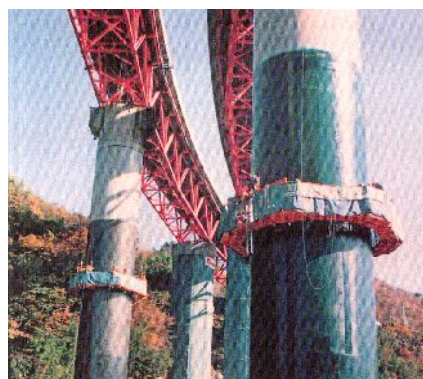
Bridge pier reinforcement
